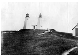
Rebuilt structure at Gurnet Point
